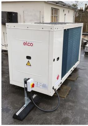
The heat pump was craned into position on the rooftop and connected to the existing heating system. Plus, thanks to the built-in protocols of the AEROTOP® unit, it was easily synchronised to the BMS to allow centralised control of the heat pump's operation.
