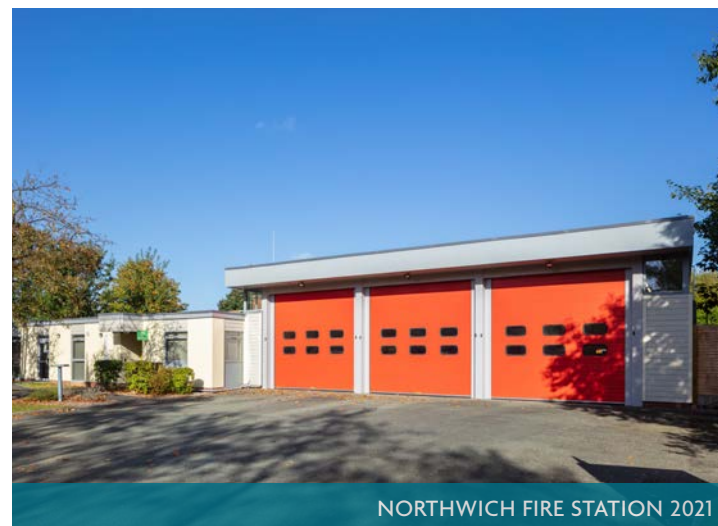
NORTHWICH FIRE STATION 2021
