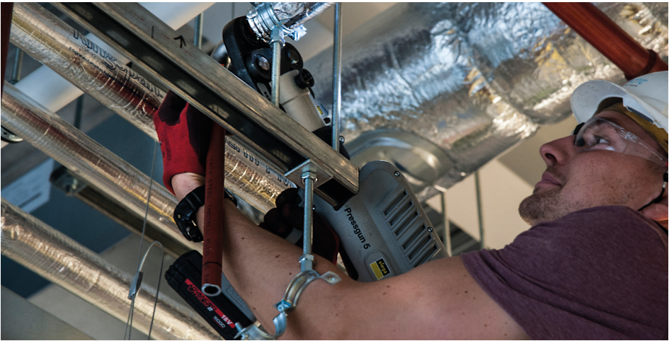
Megapress connectors are pressed easily, quickly and safely using Viega's Pressgun 5 machine.
