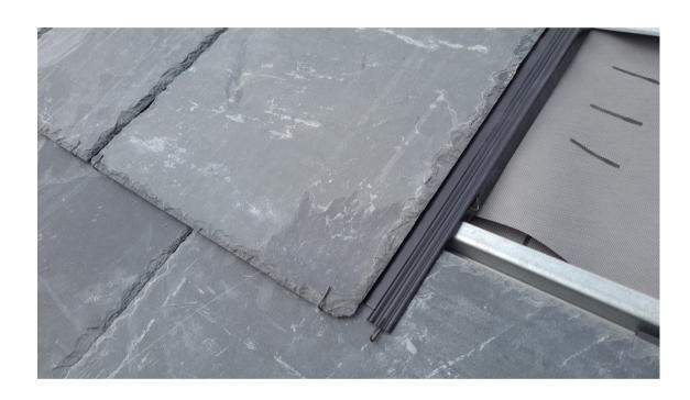
The link channels are then snap fitted to the batten to form an interlocking grid system
