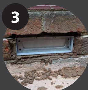
3 Start & Install AirEx device
