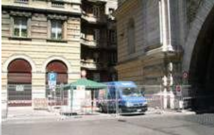
CTG working site, next to the tunnel (via del Tritone)
