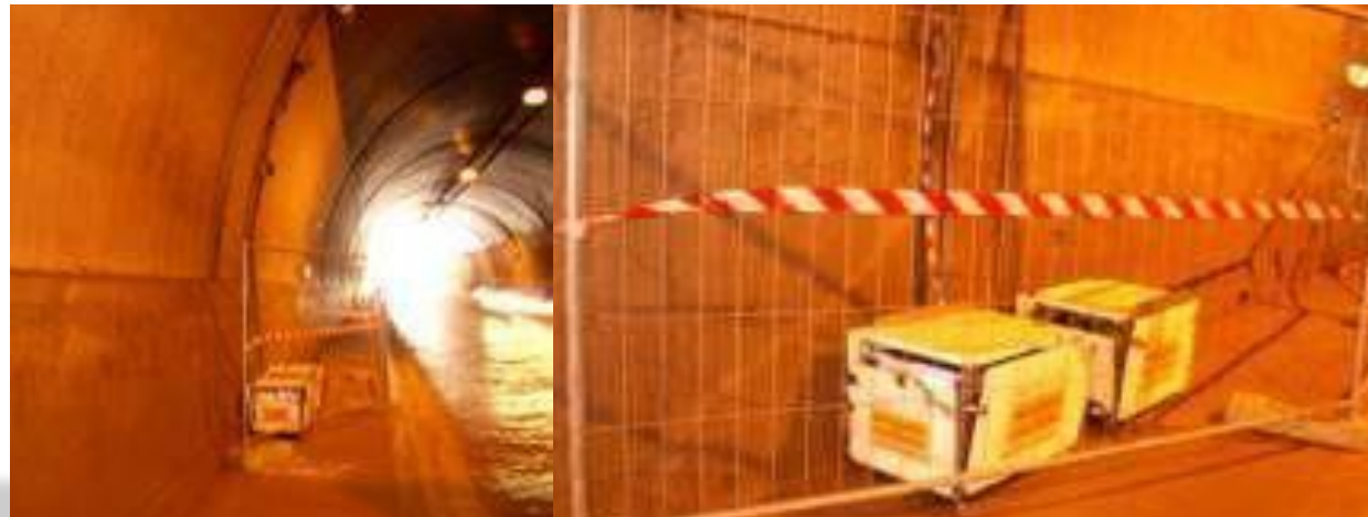
Positions of two analysers, in the centre of the tunnel (before the renovation)
